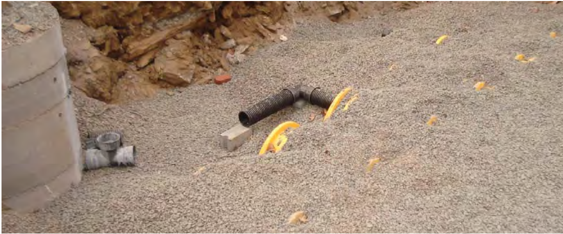
Figure 3-16: Embedment stone was placed over stormwater chambers at NYCHA's Bronx River Houses to provide structural support and additional storage volume.
