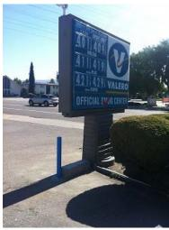
Oops... the building department missed this one. This before and after view shows an encroachment hazard along a path of travel with bottom edge of sign 40 inches above pavement. The sign was <u>not</u> lowered to less than 27 inches above pavement to comply with 2013 CBC Section 11B-307.2, instead a bollard was installed at the end of the sign and 8 inch height grouted masonry curb was installed below the sign to create detection for an individual using a cane.
