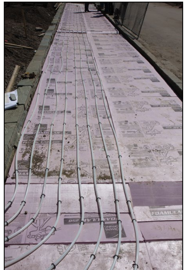
Figure 11.4 – Snow and Ice Melt Piping for a Driveway
