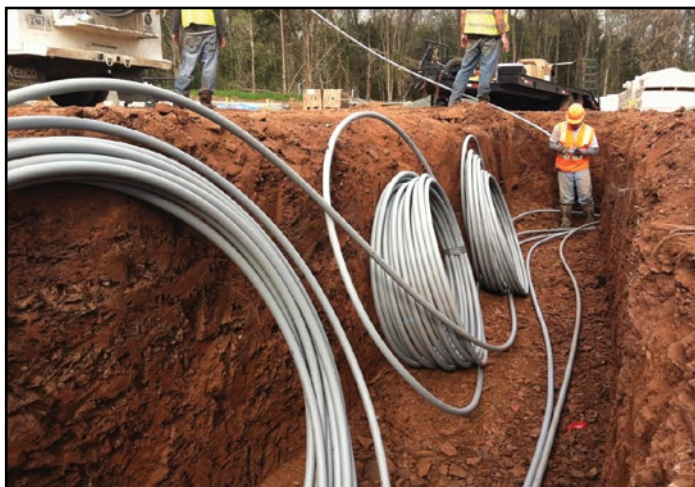
Figure 11.7 – PEX Piping in a Geothermal Application
