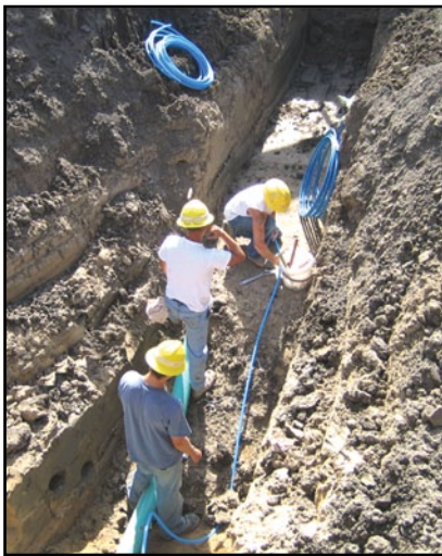
Figure 11.3 – PEX Water Service
