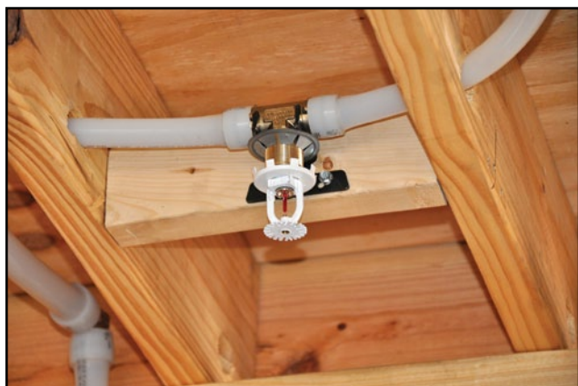
Figure 11.8 – Fire Sprinkler with PEX Piping
