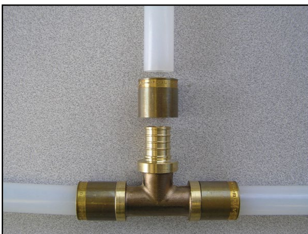
Figure 5.3 – Cold Expansion Fitting with Metal Compression Sleeve
