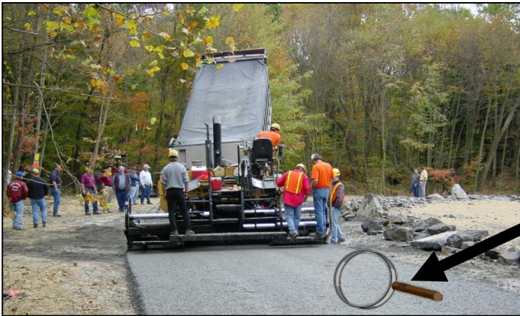
Figure 1: Placement of DSA through a paver.
