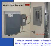
In this system the utility grid provides the back-up power and eliminates the need for batteries in the system
