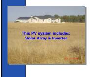
This system allows the building owner to generate and use PV power during the day and deliver excess power directly to the utility grid
