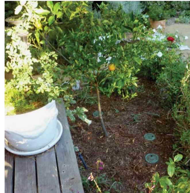
This graywater system is used to irrigate plants with similar water needs. The fruit trees and larger perennials are irrigated from the laundry machine in one “hydrozone.” Photo: Leigh Jerrard.
