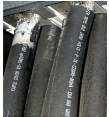
Figure 10. Do the requirements of the NEC or the NESC apply to this 650-strand DLO-type cable?
