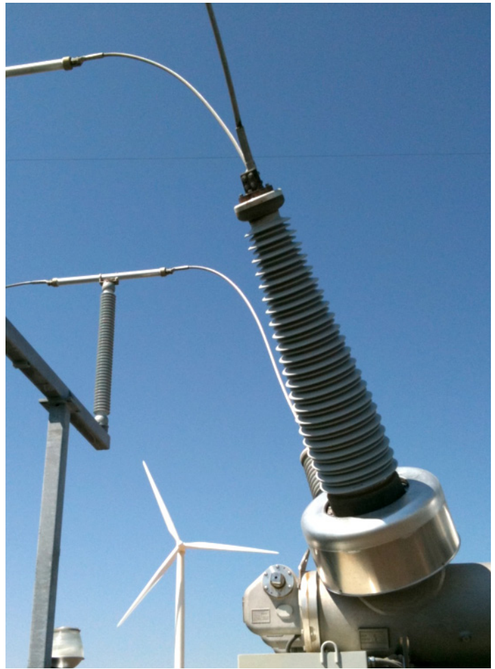
Figure 1. Voltages on a typical wind farm range from 5V dc-34.5kV ac. Available fault currents can be above 100kA. Pictured here is a 230kV output from a farm's substation to the grid.
