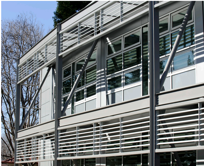
One green feature of the building is its windows, which are automated to open at night and allow fresh, cool air to enter the building. Image credit: NASA/Ames Eric James
