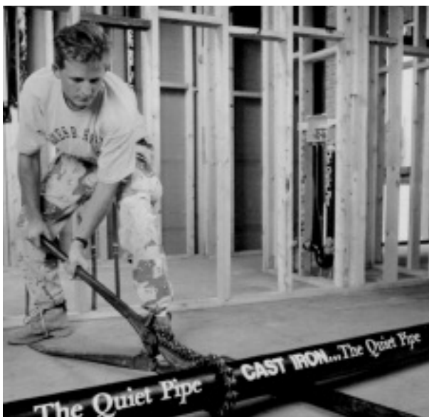
Figure 4—Assembling Hubless Cast Iron Soil Pipe Is Literally a Snap. Only Two Tools Are Required, a Pipe Cutter and Torque Wrench.
