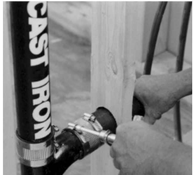
Figure 4—Assembling Hubless Cast Iron Soil Pipe Is Literally a Snap. Only Two Tools Are Required, a Pipe Cutter and Torque Wrench.
