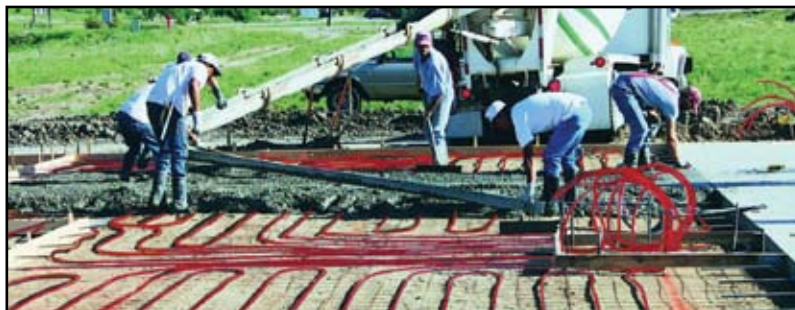
Figure 11.1 – Radiant Floor Heating Piping
